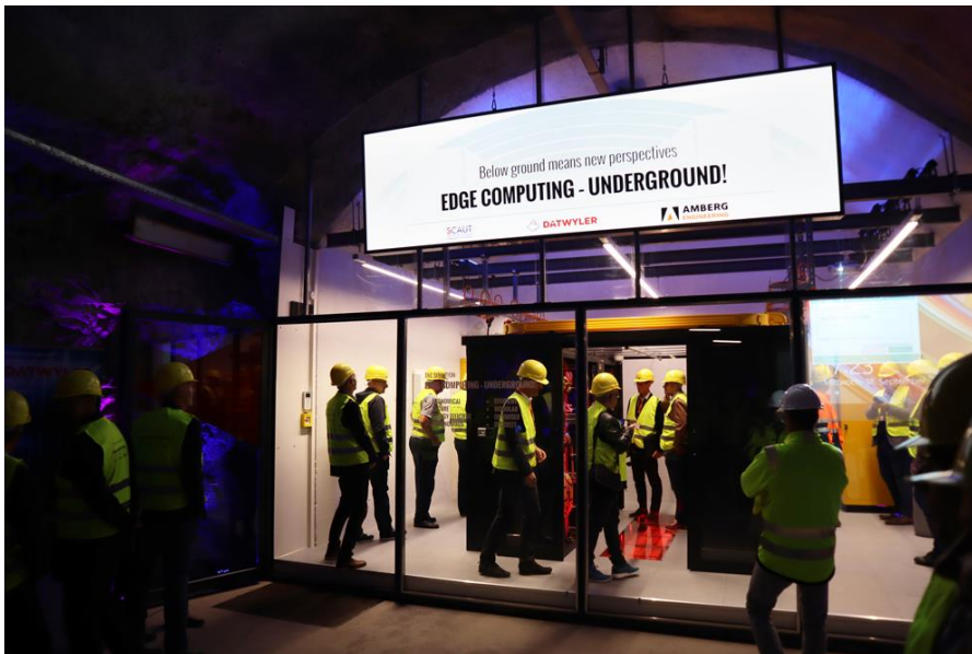
Images: Amberg Engineering Ltd. / Dätwyler Cabling Solutions Ltd.
